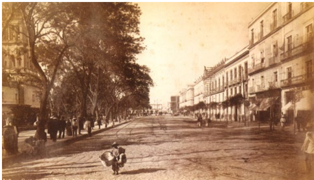
Gave & Norton, Calle del Empedradillo , ca. 1883
